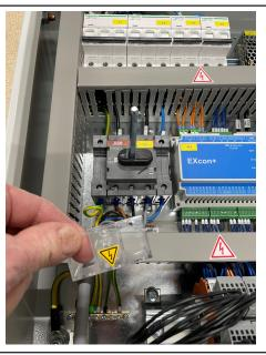
2) Finally, connect the supply voltage to the main switch.
