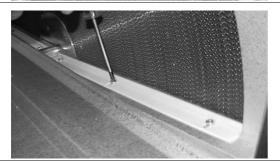
Use screws to fit the sealing strip to the blowout zone. Before finally tightening the screws, adjust the sealing strip so that the brushes touch the rotating heat exchanger.
