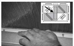
The blowout zone is placed in from the top cover against the rotor and is secured from the bottom cover. Before fully-tightening, adjust the sealing strip via the oblong screw holes, so the brushes touch the rotary heat exchanger. (If you are in any doubt about the correct distance, check the facing sealing strip).
