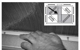
The blowout zone is placed in from the top cover against the rotor and is secured from the bottom cover. Before fully-tightening, adjust the sealing strip via the oblong screw holes, so the brushes touch the rotary heat exchanger.
