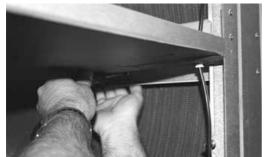
Remove the bracket with the sealing strip closest to the service door.
