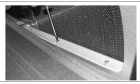
Use screws to fit the sealing strip to the blowout zone. Before finally tightening the screws, adjust the sealing strip so that the brushes touch the rotating heat exchanger.
