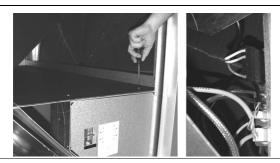
To dismantle the frequency converter, remove the screws and pull out the box.
