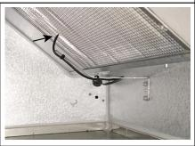
Check that the sensor T<sub>ice</sub> is correctly positioned. The sensor must protrude approx. 10 mm between the heat exchanger fins, as otherwise the sensor will not measure correctly.
