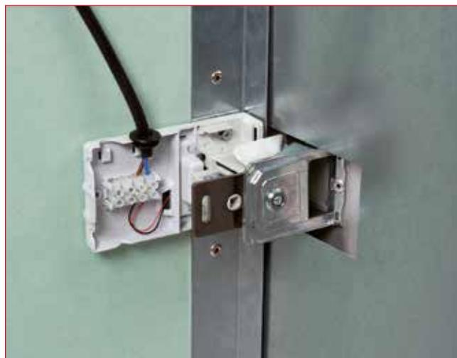
Bornier de raccordement 4 plots
